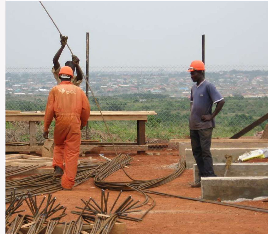
A health clinic under construction in Accra, Ghana.
